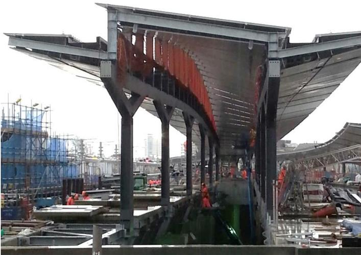
Above: This photo shows the canopies in cross section during construction. The walkable gutters, drainage columns, recesses for speakers and lights and glazed panels are visible.
