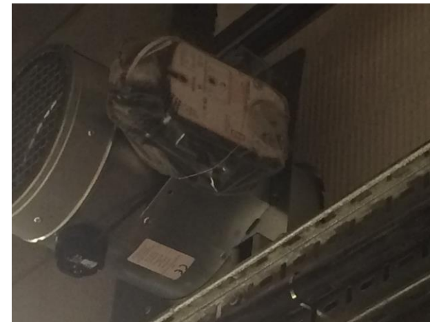
Example of fire batt installed inside the wall line.
