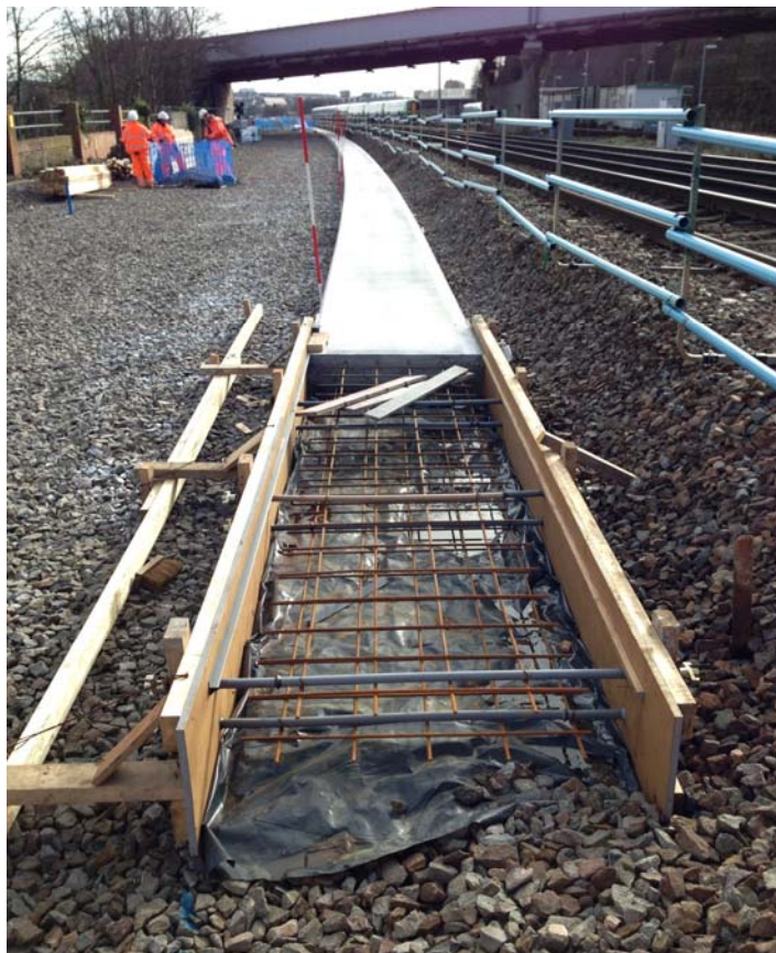
Photo 2 - Typical walkway construction at Brighton showing wooden shuttering.
