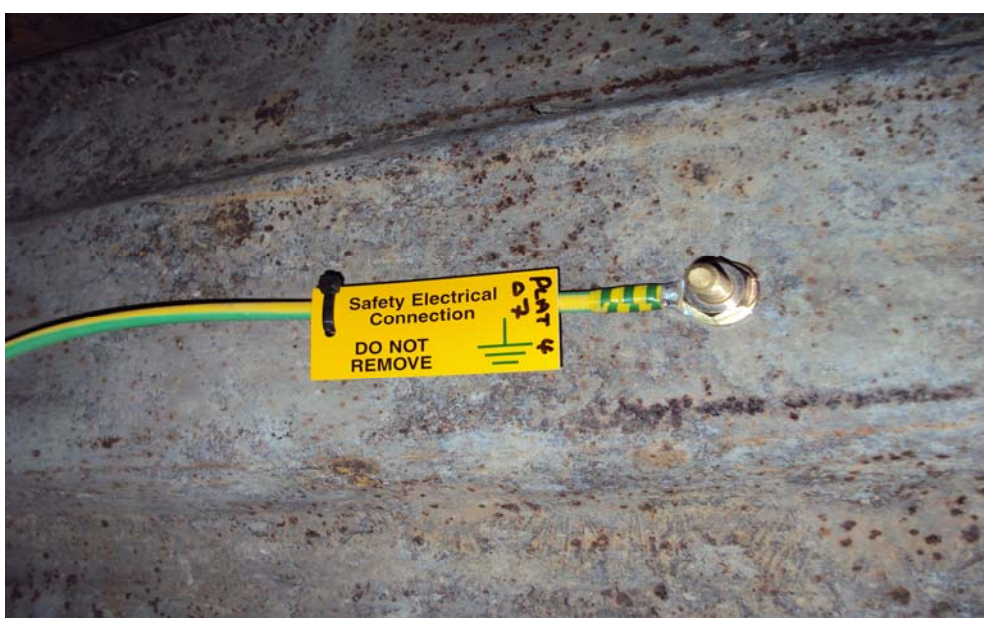
Example of Earthing wire
