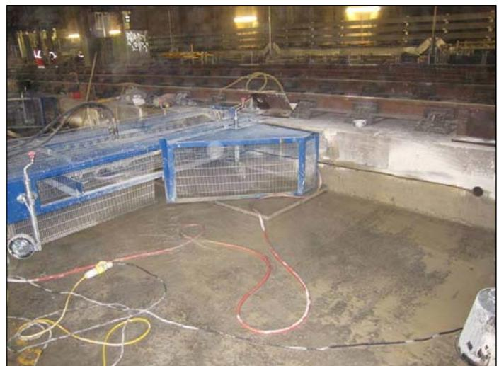
Figure 1 - Diamond Wire Cutting Rig
