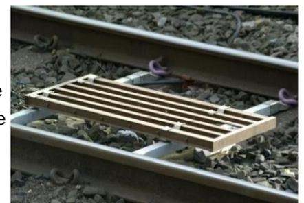
Pic 3.TPWS loop installed on tracks
