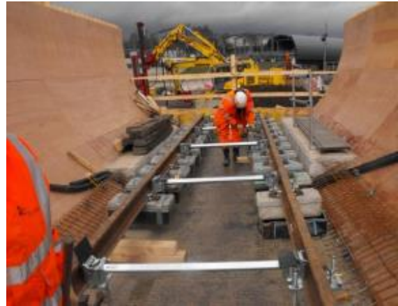
2 – Preparing to install trial track slab
