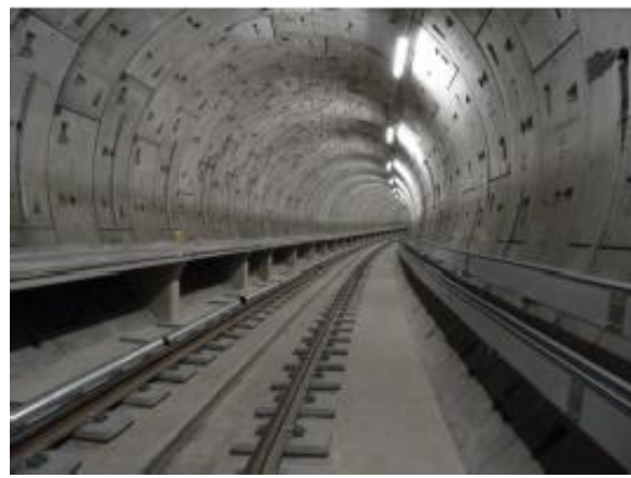
4 – As constructed track slab, walkway and CMS
