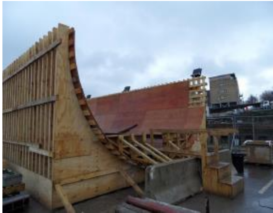
Photo 1 – Tunnel mock-up under construction (above)
