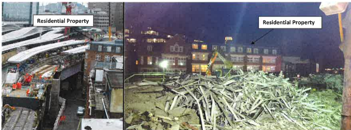
Photos showing location of residents in relation to the construction works.
