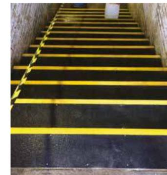
Signals and Telecoms. The steps have been smoothed out, some anti-slip laid down and some high viz paint used to highlight the steps. Staff are reminded to use the hand rail and maintain 3 points of contact at all times.
