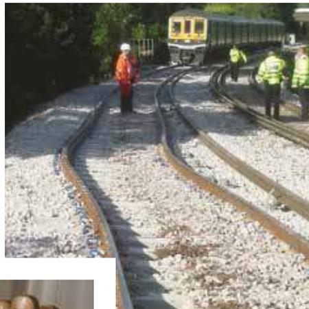
(Above) Example of buckled track through insufficient ballast on Thameslink
