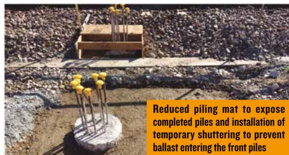
Reduced piling mat to expose completed piles and installation of temporary shuttering to prevent ballast entering the front piles
