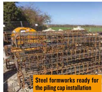
Steel formworks ready for the piling cap installation
