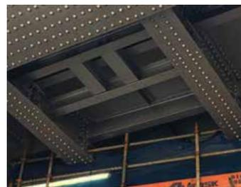
Figure 4 New trimmer beam installed
