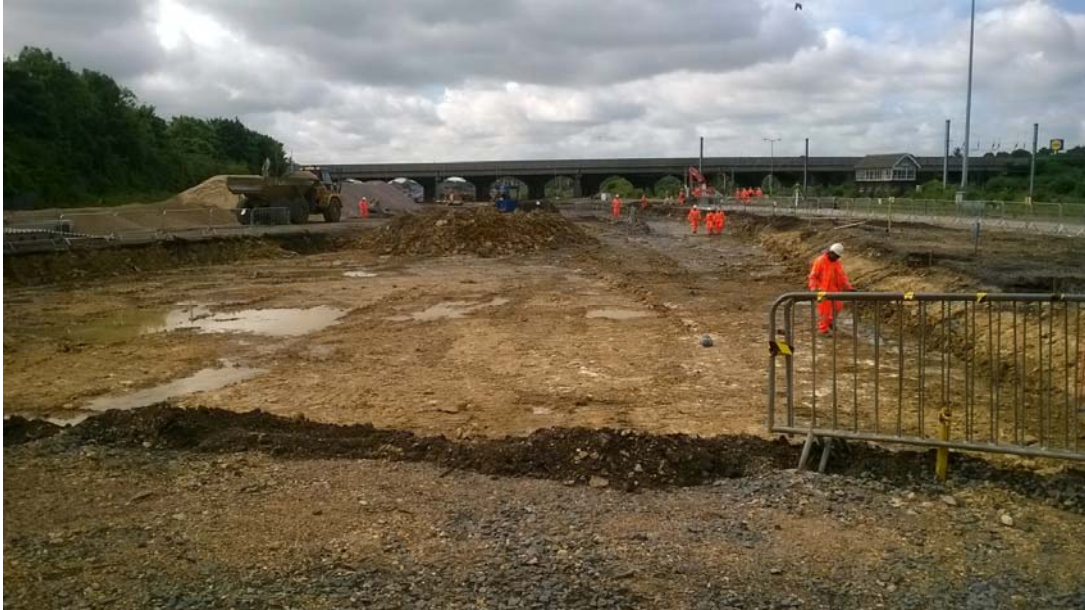
Photo 1 – Excavation works at northern end of Peterborough sidings
