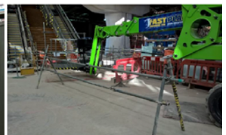
Scaffold A frames
