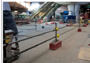
Scaffold on lollipop supports
