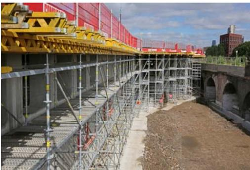
Integrated access platform runs full length of structure
