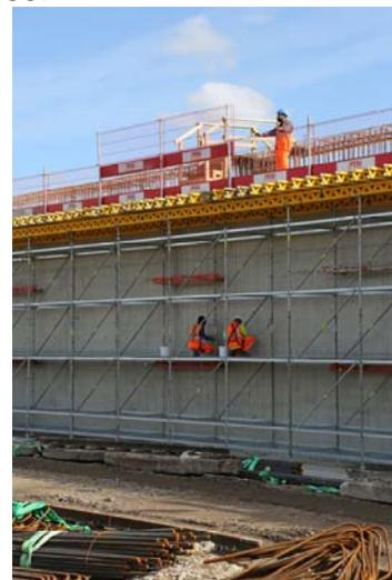
Concrete finishers working in intermediate access platform
