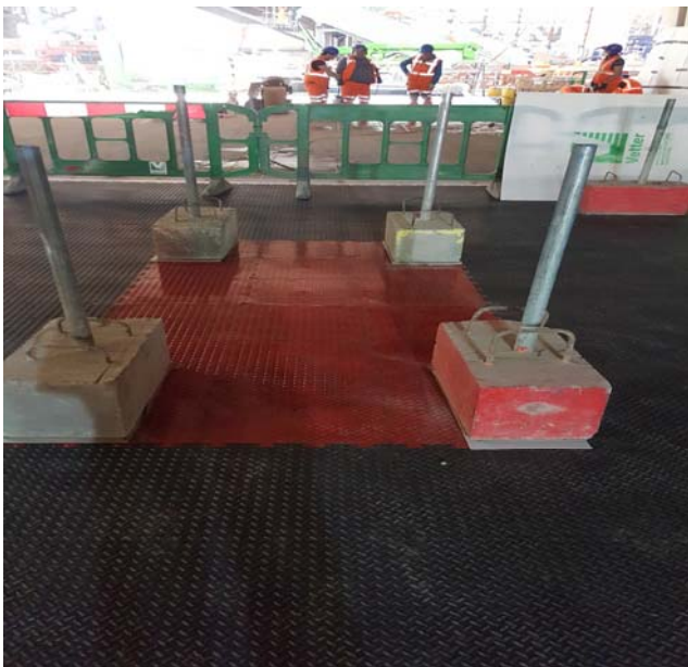
Checker plates – Red indicate pits below
