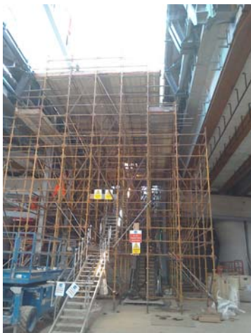
Traditional method using scaffold to inspect
